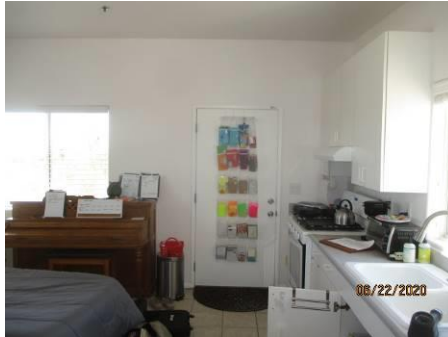
Water staining and discoloration observed under sink cabinetry.
